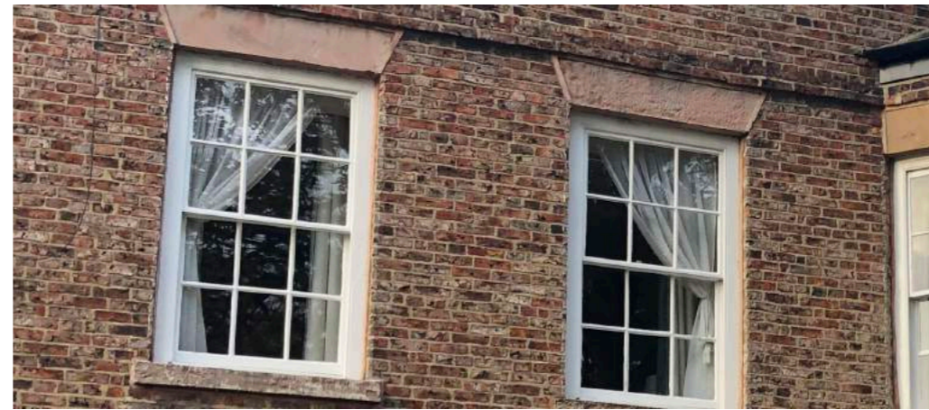
ORIGINAL SASH WINDOWS
